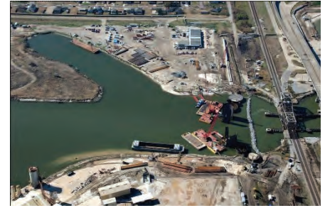
Flood gate (completed in 2012)
