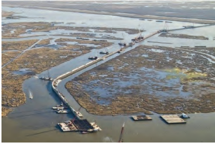
Flood walls (new walls completed in 2018)
